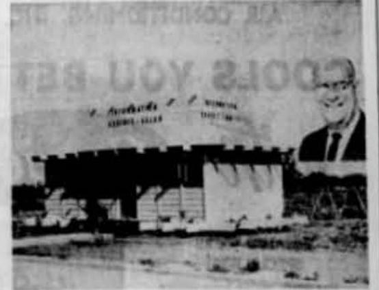
College Hills West Field Office
